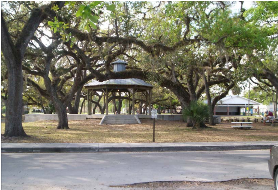
Existing Barron Park Gazebo
