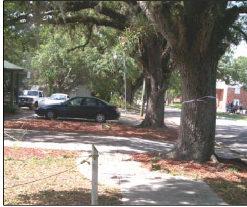
Lack of Connecting Sidewalks
