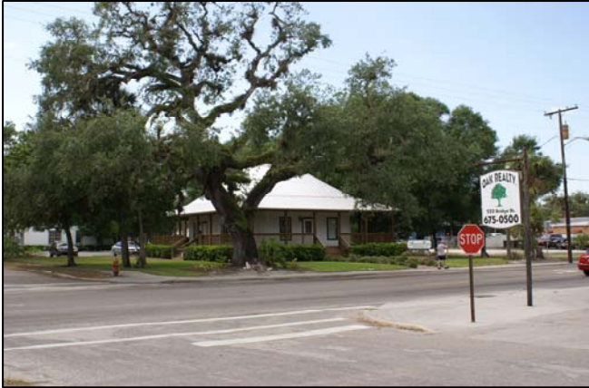
Old Florida or Cracker
